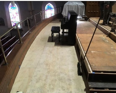
Figure 5: After the Riser Platform and Piano Platform Removed, increasing the walk-way space.
