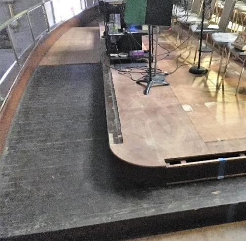
Figure 2: The Floor to Railing Height is very limited, and additional step required to access Riser Platform creating a Safety Concern.
