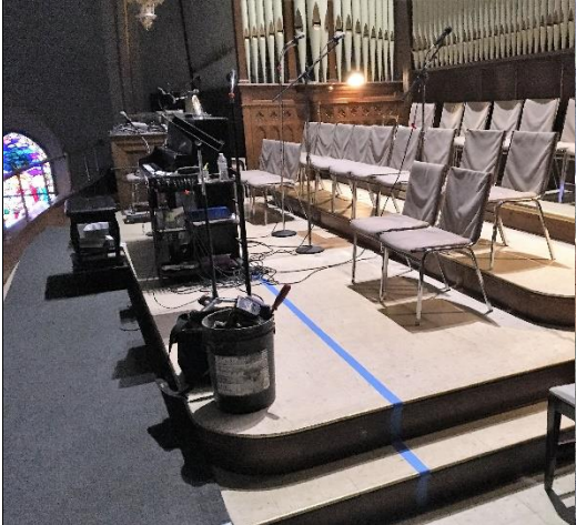
Figure 1: Blue Tape on floor indicates where the Riser Platform was to be cut to lower the floor back to the Railing. Notice Piano bench rests on a portable Platform and the limited walkway space.
